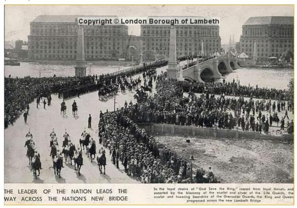
The present bridge, which has five spans and is of steel construction, extends from the site of the old abutment on the Westminster side to a point 81 feet upstream of the centre of the old Lambeth abutment. The width between the balustrades is 60 feet, there being a 36—foot roadway with 12—foot footways on each side. The balustrade is of cast-iron seated on a steel cornice and it is surmounted by cast-iron lamp standards, two on either side of the bridge in each span. There are also
